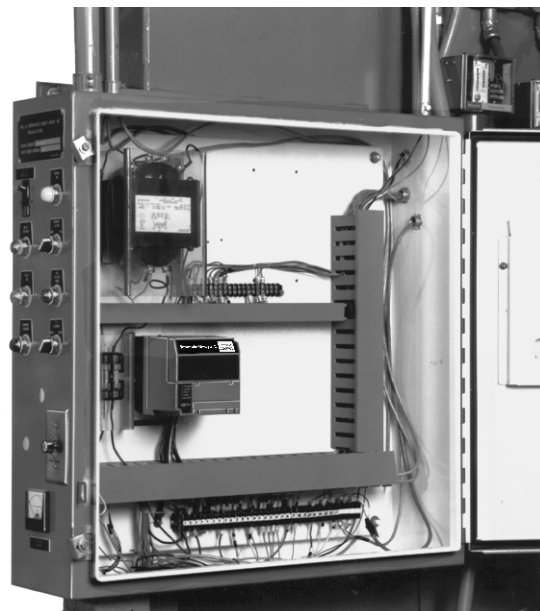
Fig. 9. Electrical panel installation.
